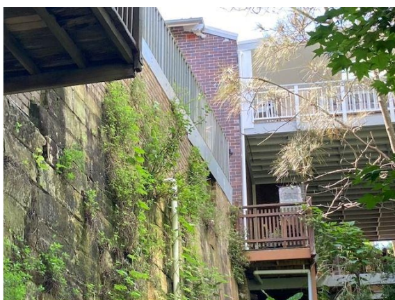
Figure 15. Partial view of the rockface and sandstone blocks forming the retaining wall running east-west through the middle of the subject site.
